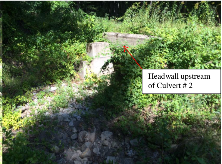
Headwall and flow path downstream of Culvert #2
